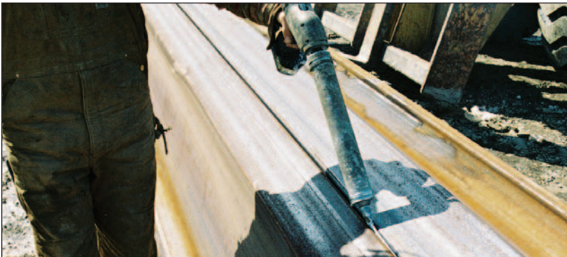
Swellseal® WA applied with caulk gun
