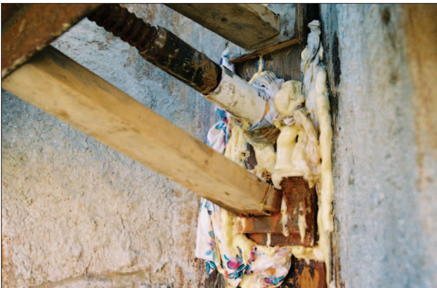
Tieback sealed with HYDRO ACTIVE® CUT
