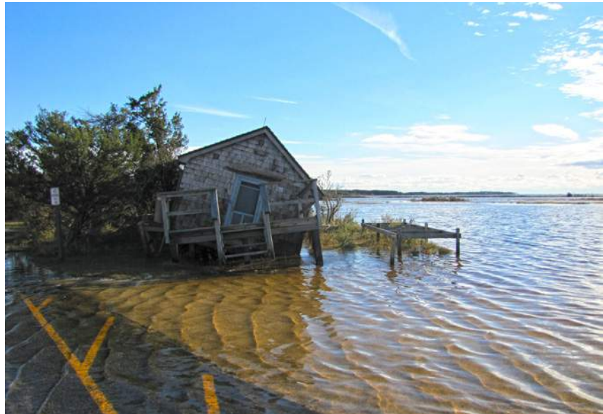
Assateague Historic National Seashore subject to considerable flooding, erosion, and infrastructure damage following Hurricane Sandy in 2012.
