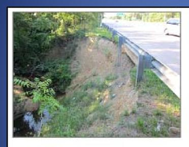
July 2010 – Erosion has progressed significantly. Photos on the right show that Moravia Road is now being undermined.
