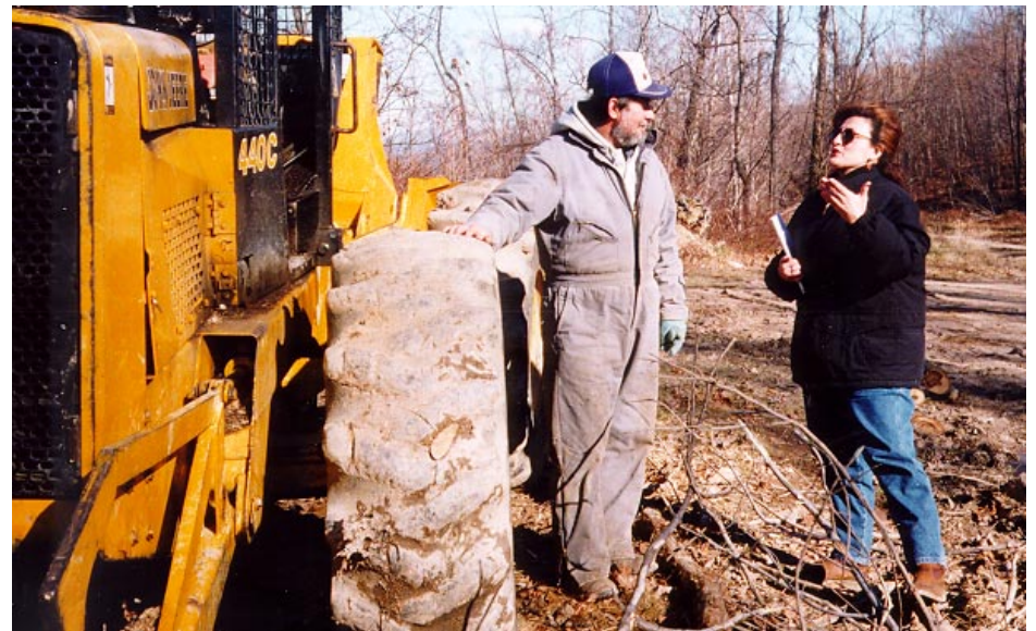
MDE inspector Lisa Trujillo visits a local construction site.
