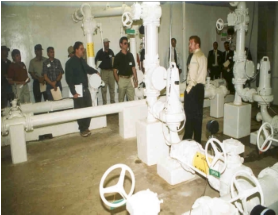
Tour members review the intricate network of pipes in the underground pumphouse at the Mt. Airy Wastewater Treatment Plant.
