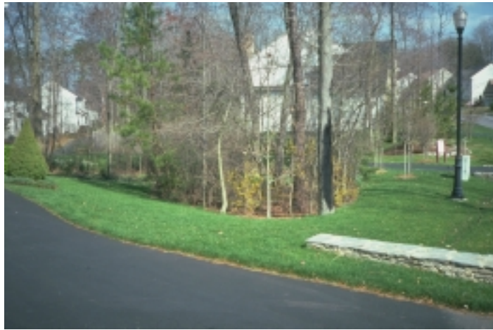
Bio-retention stormwater projects like the one above are cataloged in a new MDE database accessible on the web. The landscape is designed such that stormwater runoff collects in shallow depressions before filtering through fabricated planting soil media.
