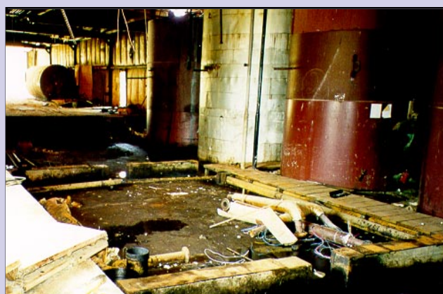
Above, a before shot of a creosote contaminated work pit at Eastern Maryland Wood Treating Company that once held a wood treatment cylinder and several large work tanks filled with tar-like creosote. Right, the same pit after final sealing of the structure with concrete.
