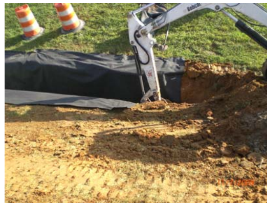
Figure 3-6 Infiltration Trench 020193 In-Kind Replacement
