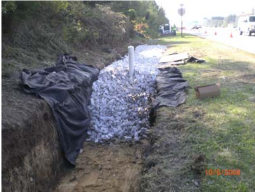
Figure 3-6 Infiltration Trench 020193 In-Kind Replacement
