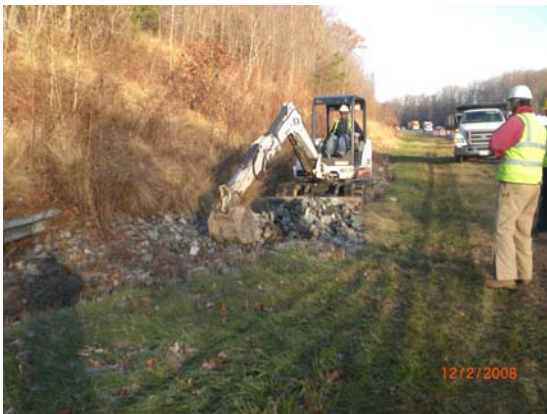
Figure 3-2 BMP 020186 – Removal of Sediment from Infiltration Trench
