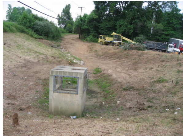
Figure 3-3 Inflow Channel Stabilization (BMP130292) - during construction
