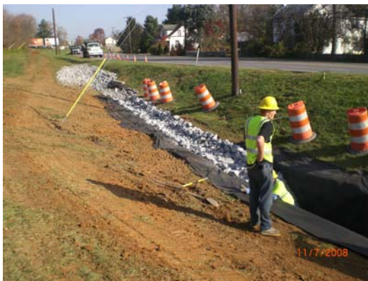
Figure 3-6 Infiltration Trench 020193 In-Kind Replacement
