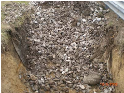
Figure 3-5 Excavation of Infiltration Trench 020191
