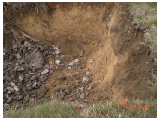
Figure 3-5 Excavation of Infiltration Trench 020191
