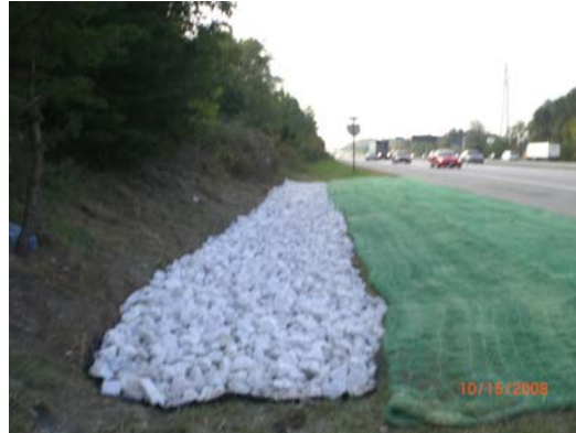
Figure 3-6 Infiltration Trench 020193 In-Kind Replacement
