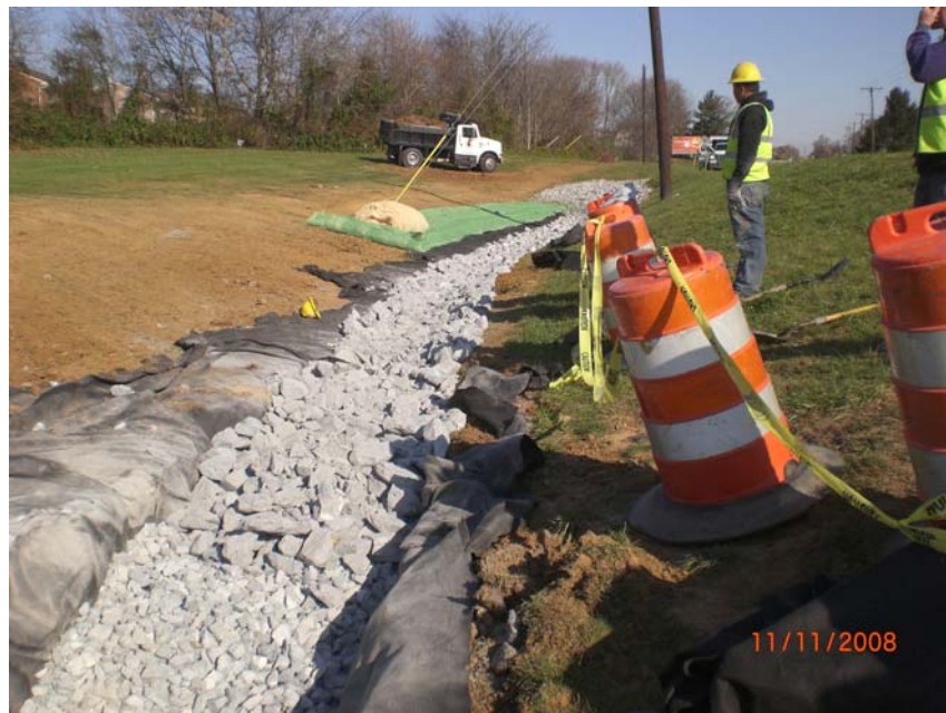
Figure 3-7 Infiltration Trench 210013 In-Kind Replacement
