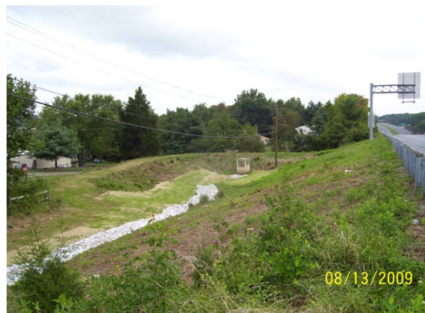
Figure 3-4 Inflow Channel Stabilization (BMP13007) – After Construction
