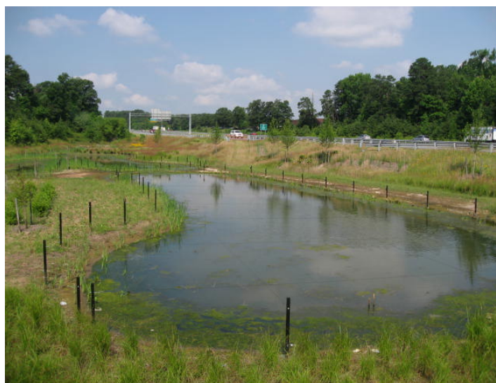
Figure 3-9 Functional Enhancement of Infiltration Basin at MD 100 into Shallow Wetland (BMP 020120)
