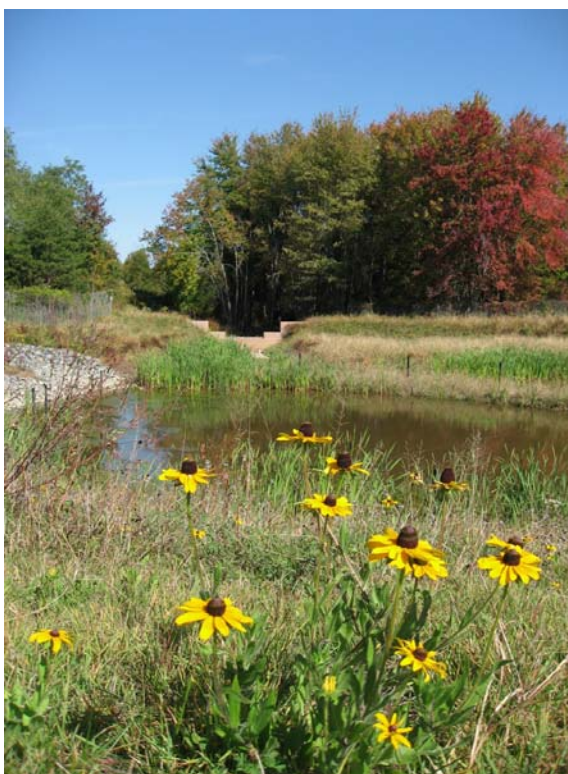
Figure 3-12 Reconstruction of Failed Infiltration Basin at MD 100 into Micro-pool Extended Detention Pond (BMP 020111)
