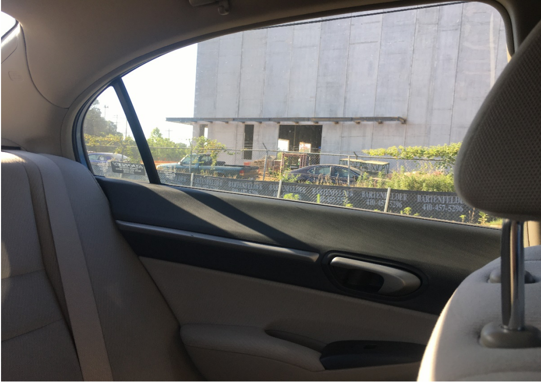
Active Construction In Section 1
