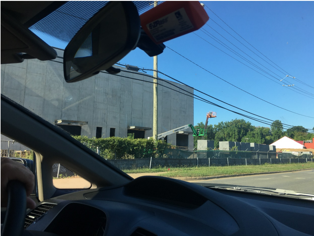
Active Construction in Section 1
