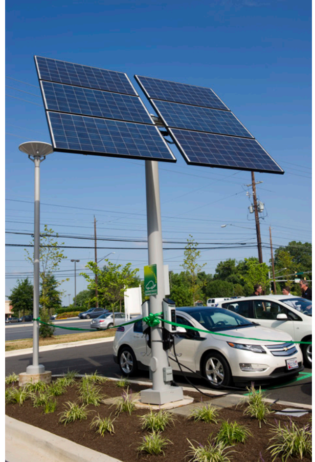
Tracking solar array to charge electric cars.
