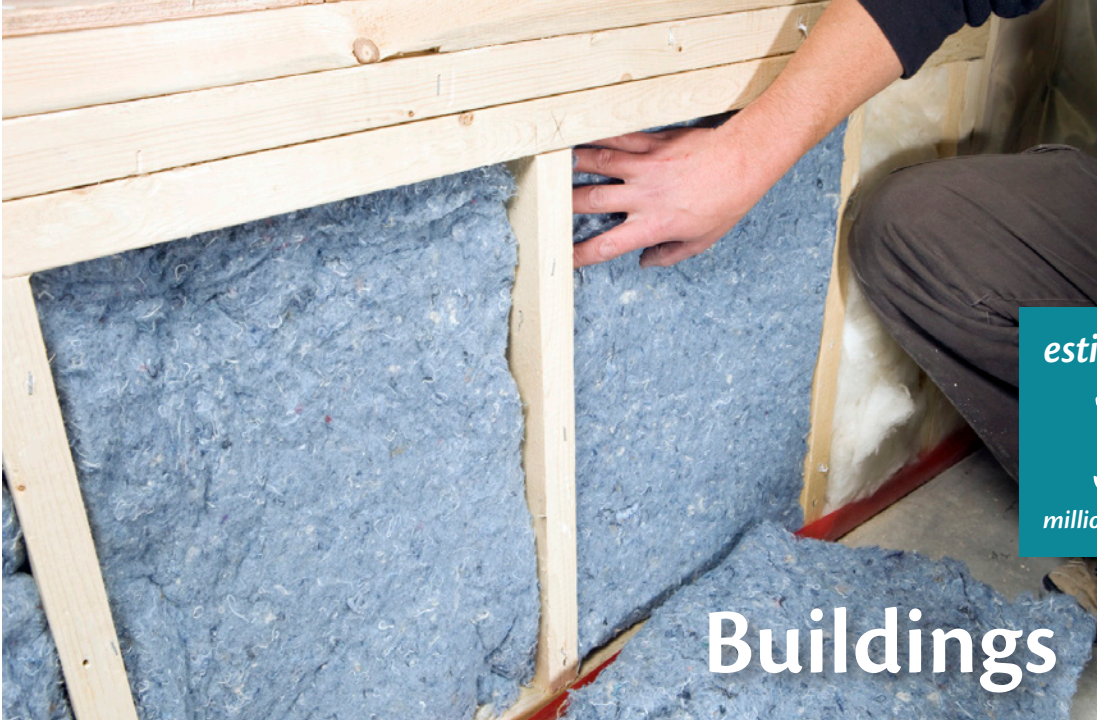
A worker installing recycled blue jean denim insulation.
