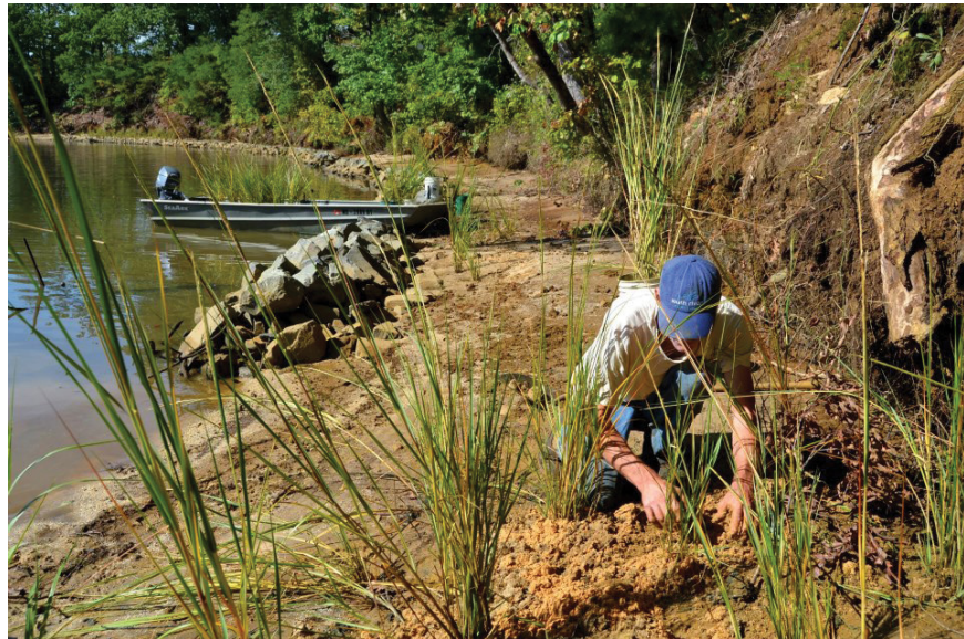
Living shoreline project on Church Creek will help to stabilize the shoreline and allow swamp, shoreline, and floodplain forest species to migrate to higher elevations.
