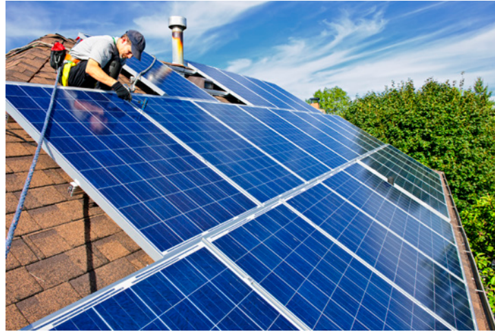
Reducing Maryland's GHG emissions will also create new jobs, such as installing solar panels on residential buildings.
