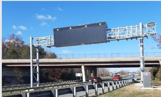
EB MD 175, west of I-95 Direction Specific DMS Signs
