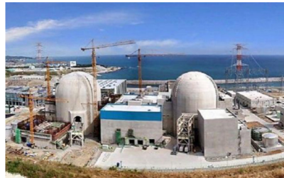
Gen III nuclear built with best project management practices (UAE-KEPCO reactors delivered at $3,000/kw)
