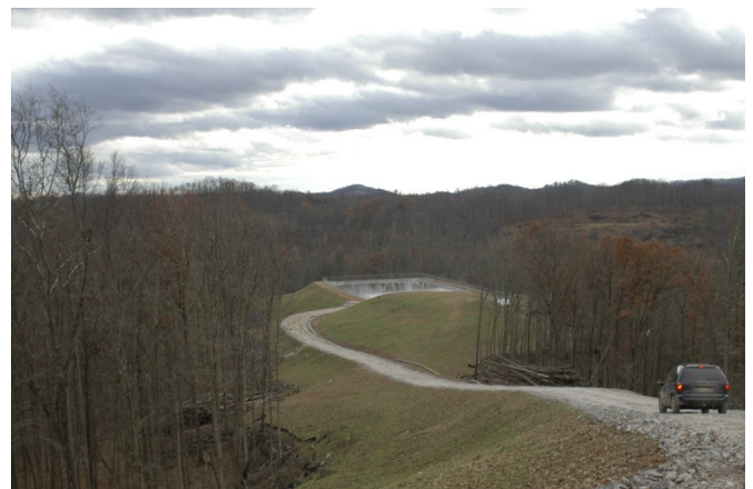
Fig. 2. Road and storage pond constructed on surface owner's property.
