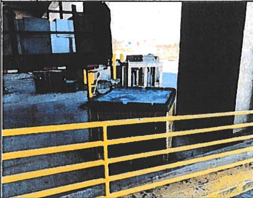
Photo #15: Spill kit within the loading/unloading area.
