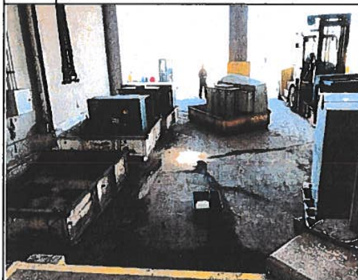
Photo #10: Transformer storage within the loading/unloading bays.
