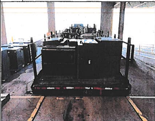
Photo #17: Transformers drained and loaded onto transport for disposal.
