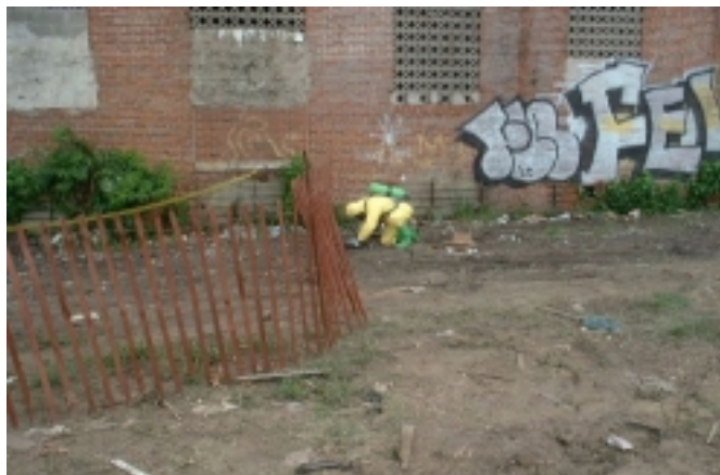
Sampling activities at the Better Buildings Warehouse located on Heath Street in Baltimore City.
