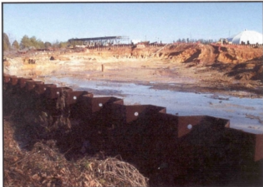
BEFORE: Soil excavation during Winter 2000 in the area of a former waste disposal pit for wood treatment chemicals.
