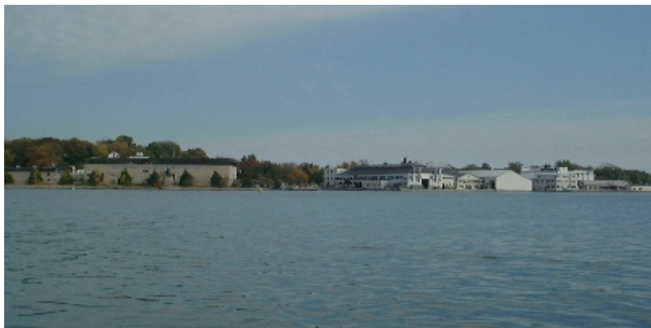
View of Naval Surface Warfare Center from the Severn River.
