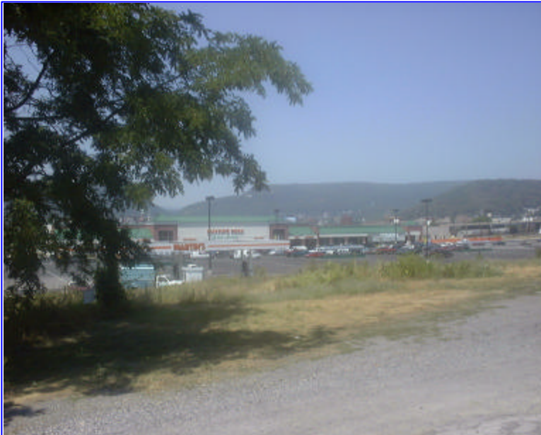
Redeveloped property following implementation of the Voluntary Cleanup Program response action plan.
