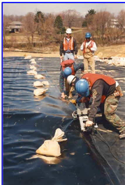
Workers cap the old base landfill at Bainbridge.
