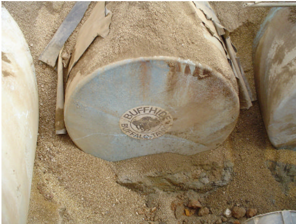
Photo 3 - View of south end of 8K UST.
