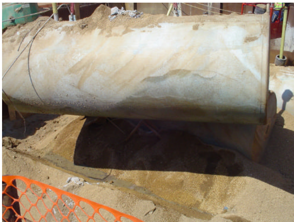
Photo 6 - View of 8K2 UST removal facing west.
