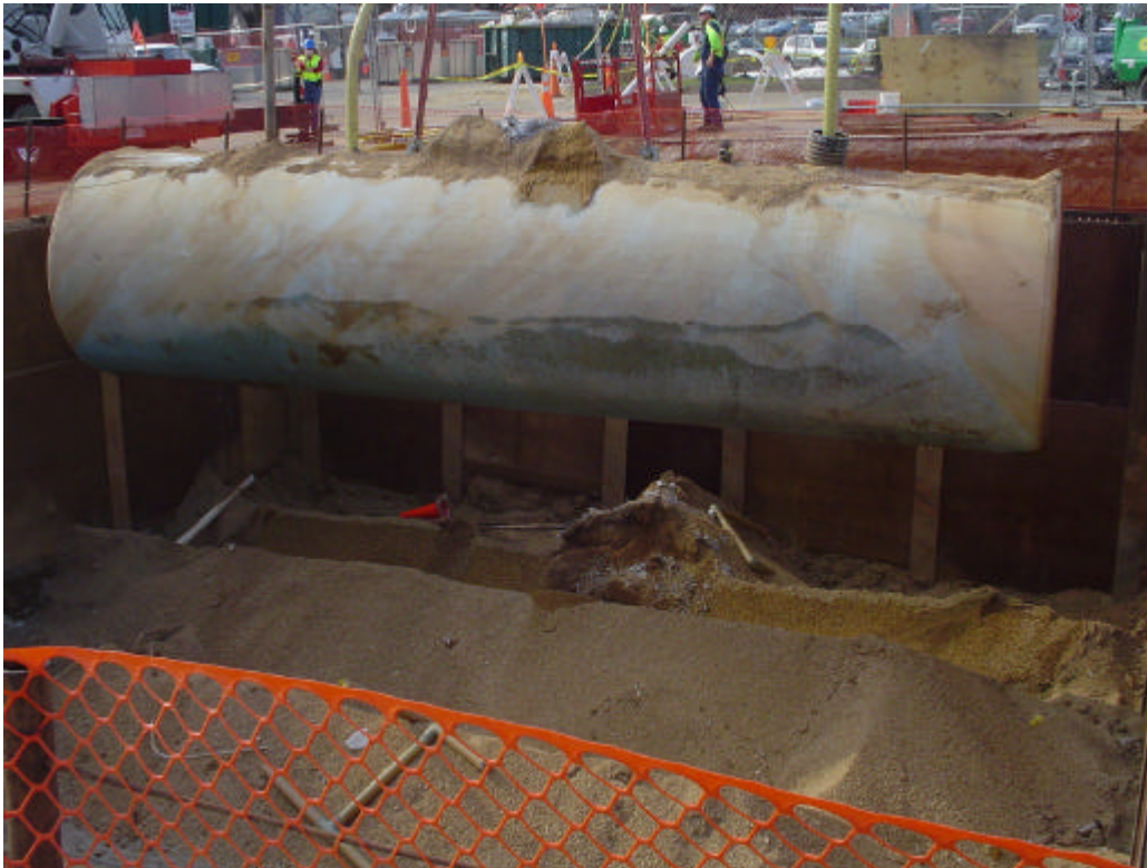
Photo 8 - View of 12K UST removal facing west.
