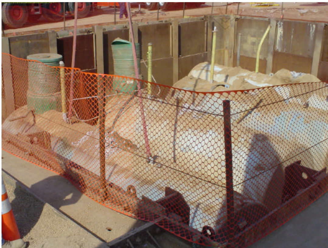
Photo 4 - View of uncovered USTs. 10K UST in foreground.
