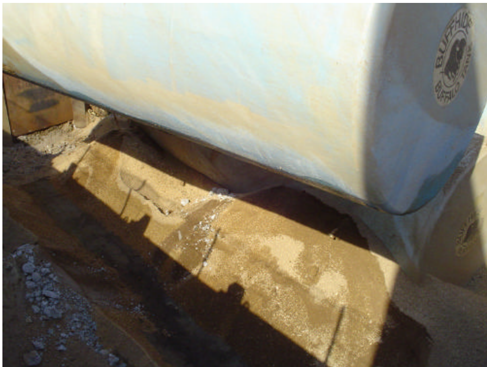
Photo 5 - View of 10K UST removal facing west.
