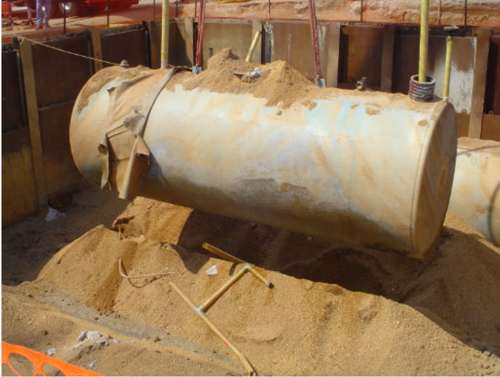
Photo 7 - View of 8K UST removal facing west.
