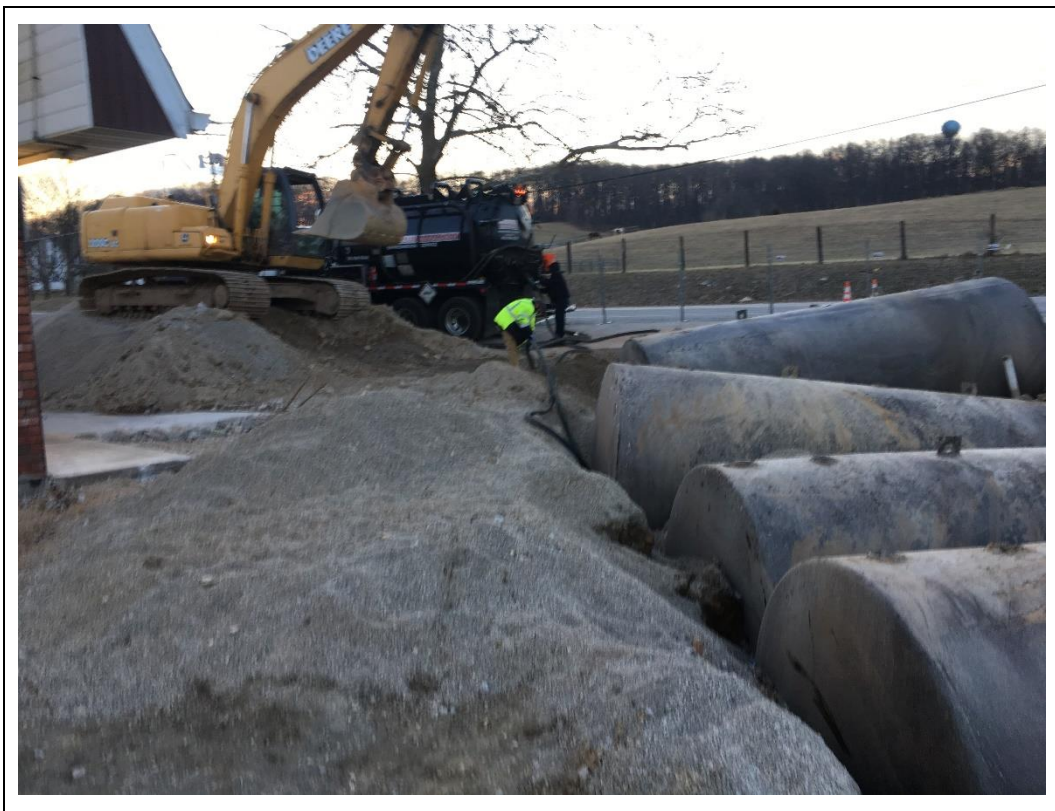
Photograph 2: View of the vacuum truck cleaning the tanks.
