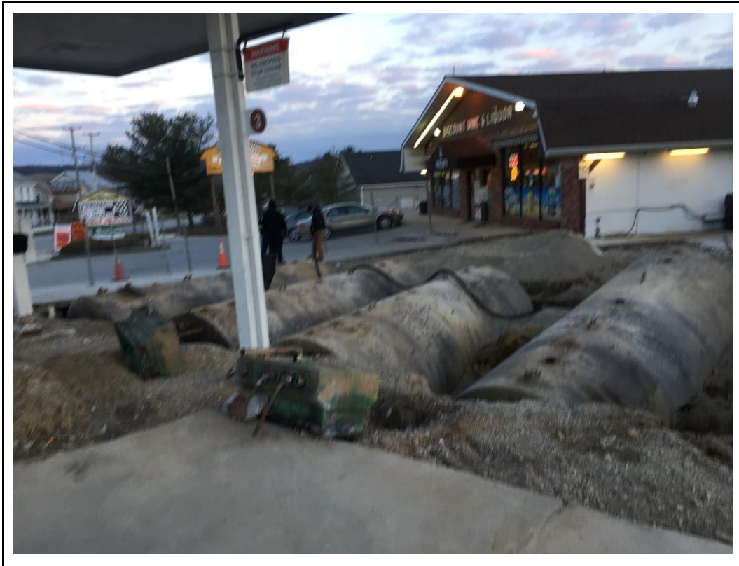
Photograph 1: View of the USTs still in the ground and uncovered.
