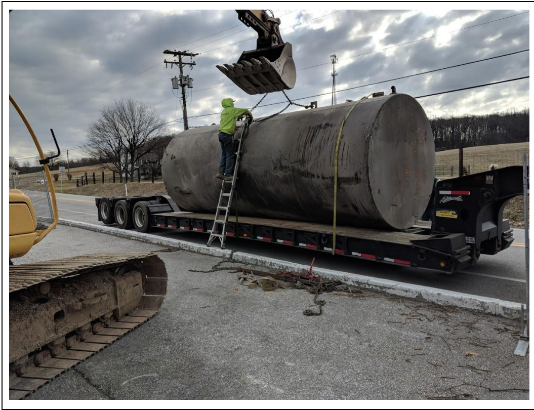
Photograph 5: View of the UST being loaded onto a truck for offsite disposal.
