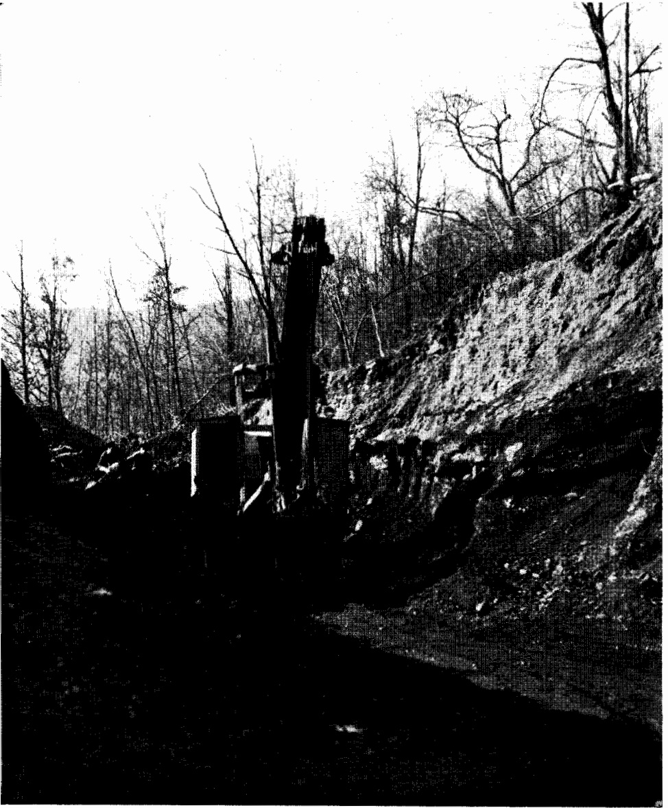
Scene of fatal accident to Charles Preston, employed at strip pit operated by Russell Mining Company, opposite Knapp's Meadow, Lonaconing, Allegany County, November 13, 1945.
