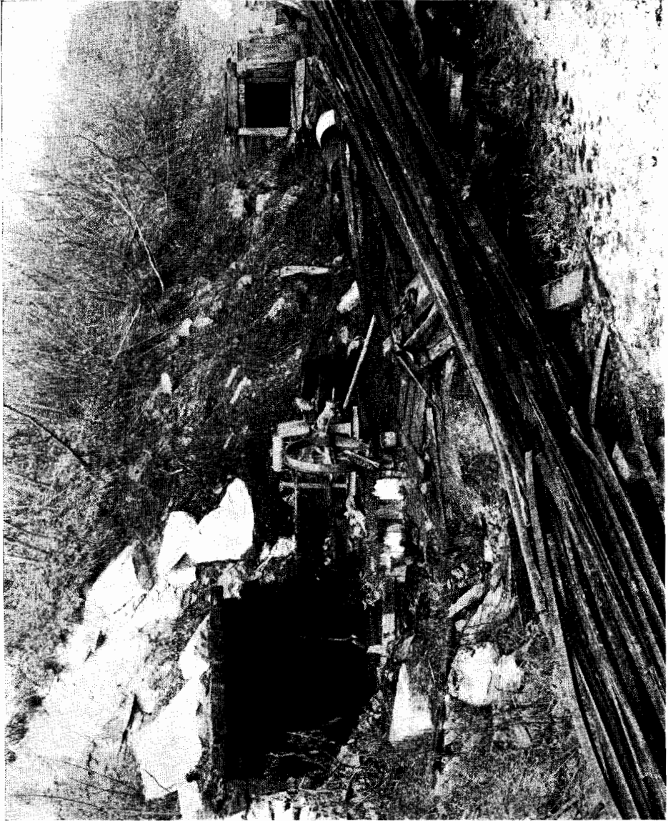
Milt No. 1 Mine showing ventilating fan after fire.
