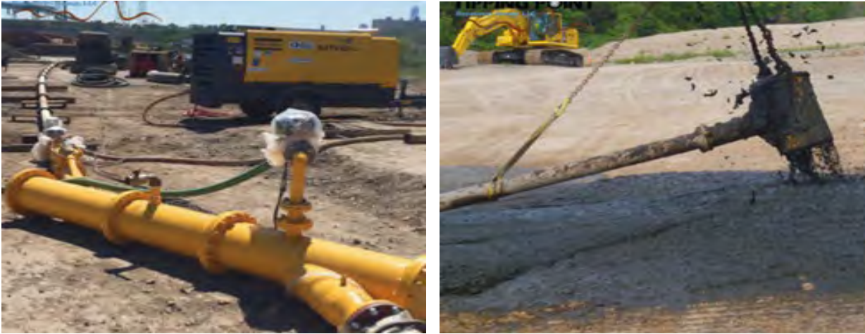
Images: Tipping Point Pneumatic Flow Tube Mixing Apparatus Producing Flowable Fill
