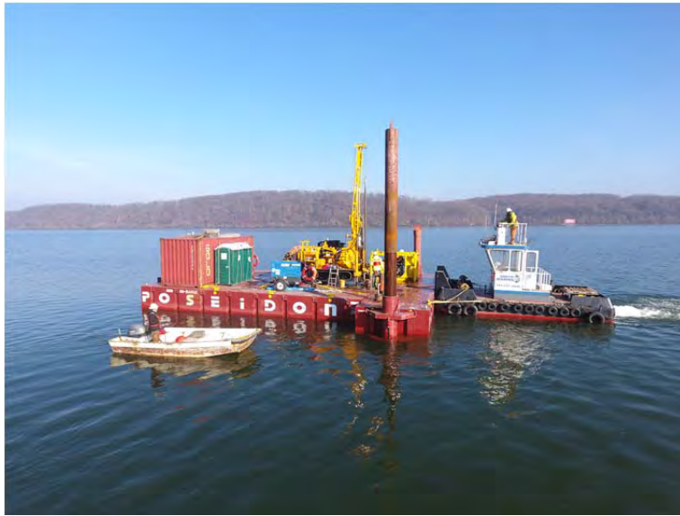
Aerial Image of Coring Operations
