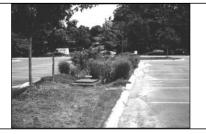
Figure 10 - Parking Lot Island Turned into Bioretention
