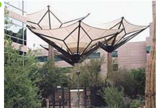
Figure 3-4. Rainwater Harvesting Shade Structure, Credit: Forgotten Rain LLC.
