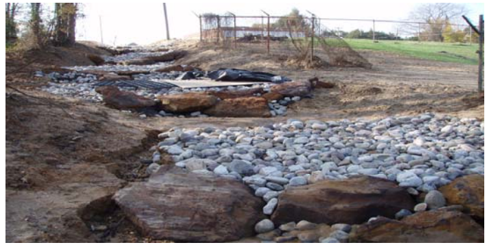
Coastal Plain Outfall (After)
