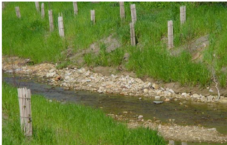
Figure 8. Less than one year after Baltimore County's Spring Branch Phase II stream restoration project graded the stream bank in this stream segment to reduce slope, the trees planted in the riparian area are still protected by tree shelters made from bamboo laced together with twine. These shelters are designed reduce animal damage to the saplings for a several year period and then naturally fall apart and decompose. (Photograph was taken at the down-stream end of the project at Dulaney Valley Road by the MDE TMDL Implementation Division).
