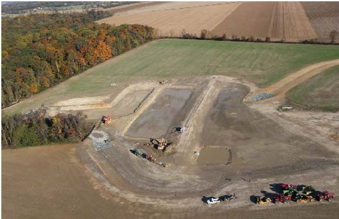
Figure 19. The Crawford Treatment Wetland is an innovative vertical flow treatment wetland being constructed downstream from a concentrated animal feeding operation (CAFO). It is designed to capture sediment and remove nutrients before directing treated water to the natural stream. The practice will be the first of its kind to capture and treat both surface stormwater from the CAFO and groundwater from surrounding crop fields. Funding is provided by the National Fish and Wildlife Foundation and Maryland’s Chesapeake Bay Trust and Maryland’s Chesapeake and Atlantic Coastal Bays Trust Fund. (photo provided by the Sassafras River Association.)
