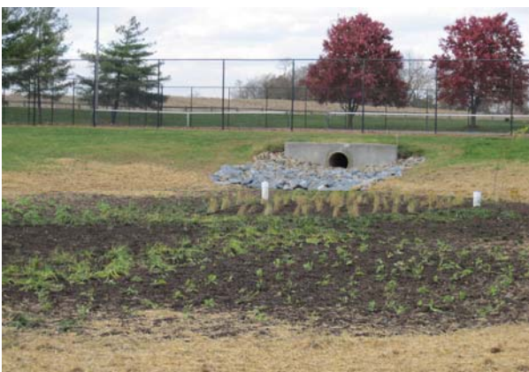
Figure 17. In 2013, Frederick County constructed a bioretention BMP in the County's Urbana Community Park to treat stormwater runoff from about 6.4 acres of the park, parking lots and roads. The 319(h) Grant provided funding assistance for the project. The BMP includes an under drain, that could be seen during construction (top). In November 2013 shortly after project completion (bottom), the new plantings are ready to play their part in helping to intercept runoff. (Map and photos are courtesy of Frederick County.)
