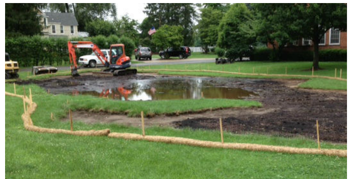
Figure 13. In 2012, Queen Anne’s County Dept. of Public Works employees initiated work to retrofit the County Board of Education building in Centreville with stormwater infiltration capabilities. Portions of the project received funding assistance from the 319(h) Grant (FFY11 #11). (above, photo by Queen Anne’s Co.) In September 2013 the County Dept. hosted MDE and EPA at an on-site review of the project’s bioretention / rain garden area in the front of the Board of Education building. At the time of the visit, vegetation in the project area was still in the early stages of growth. (left, photo by MDE)
