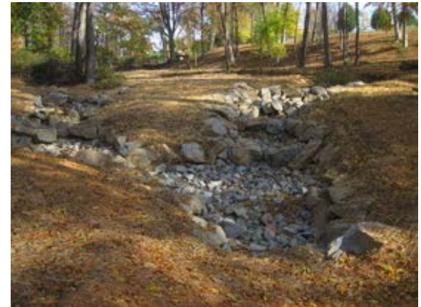
Figure 21. In 2013, the Budds Landing ravine stabilization project was constructed (left) thru the efforts of the Sassafras River Association in the headwaters of Coppin Creek in the upper Sassafras River watershed. The project area receives stormwater runoff from about 150 acres of mixed low density residential and pasture lands. The completed 1600 linear foot project (right) includes regenerative stormwater conveyance cells, rock grade control step pools, coir fiber logs and live fascines to help slow runoff and promote infiltration. To help pay for the project, the SRA received a $170,864 grant from Chesapeake and Atlantic Coastal Bays Trust Fund. (Photos are by the Sassafras River Association.)
