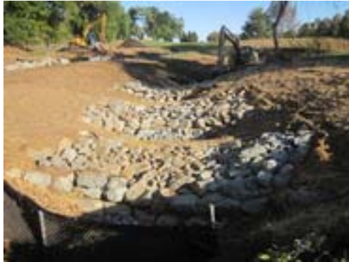
Figure 21. In 2013, the Budds Landing ravine stabilization project was constructed (left) thru the efforts of the Sassafras River Association in the headwaters of Coppin Creek in the upper Sassafras River watershed. The project area receives stormwater runoff from about 150 acres of mixed low density residential and pasture lands. The completed 1600 linear foot project (right) includes regenerative stormwater conveyance cells, rock grade control step pools, coir fiber logs and live fascines to help slow runoff and promote infiltration. To help pay for the project, the SRA received a $170,864 grant from Chesapeake and Atlantic Coastal Bays Trust Fund. (Photos are by the Sassafras River Association.)
