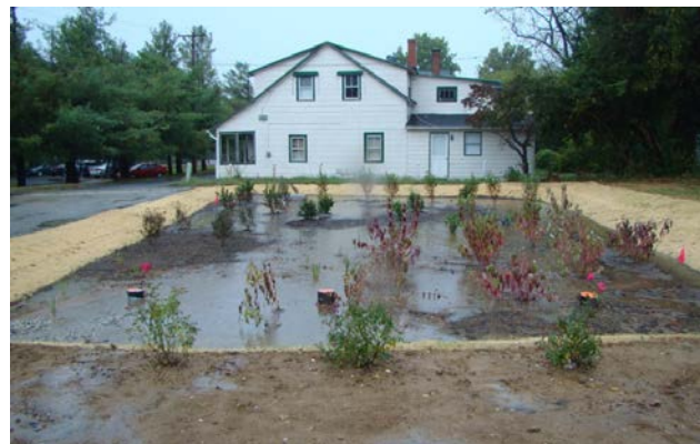
Figure 11. Adjacent to Powell Street in Centreville, part of an asphalt parking lot was converted to a stormwater infiltration area in 2013 as part of a 319(h) Grant project that continued thru 2014. The area receives runoff from an impervious area of parking and rooftops including private commercial businesses and the local fire department. (photos courtesy of the Town of Centreville)
