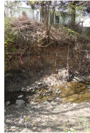
Figure 16. Scotts Level Branch between Allenswood and McDonogh Roads had significant stream bank erosion and there was little connection to the floodplain (photos left and right). Baltimore County’s watershed plan targeted this area for restoration, which was completed in 2014. (Photos courtesy of Baltimore County)
