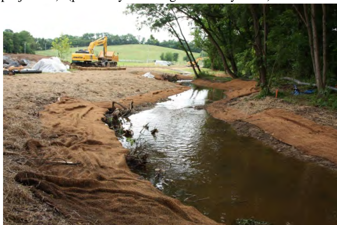
Figure 7. Stream restoration construction long Little Antietam Creek took place in 2016 (below left). Construction was completed late in 2016 (belowright). The restoration was funded in part by two the 319(h) Grant in FFY2015 project #7). (photos by Washington County SCD).
