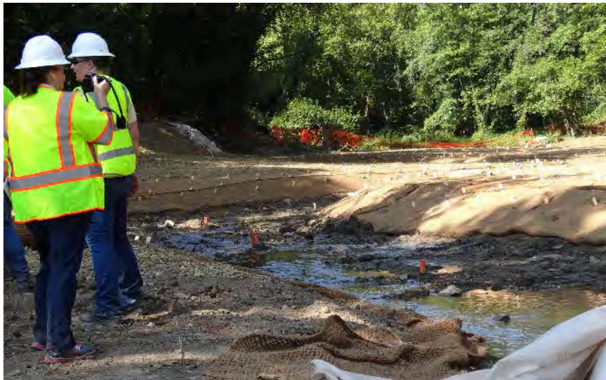
Figure 3. Baltimore County Dept. of Environmental Protection and Sustainability hosted staff from EPA Region 3 and MDE at their Herring Run stream restoration project at the County’s Overlook Park in September 2017. The photo shows a section of Herring Run that is being stabilized prior to final vegetative stabilization. This area, including the stream bed, banks and floodplain, has been reshaped to create a more-natural, stable system. The project is funded in part by 319(h) Grant FFY2014 funds. (photo by MDE)
