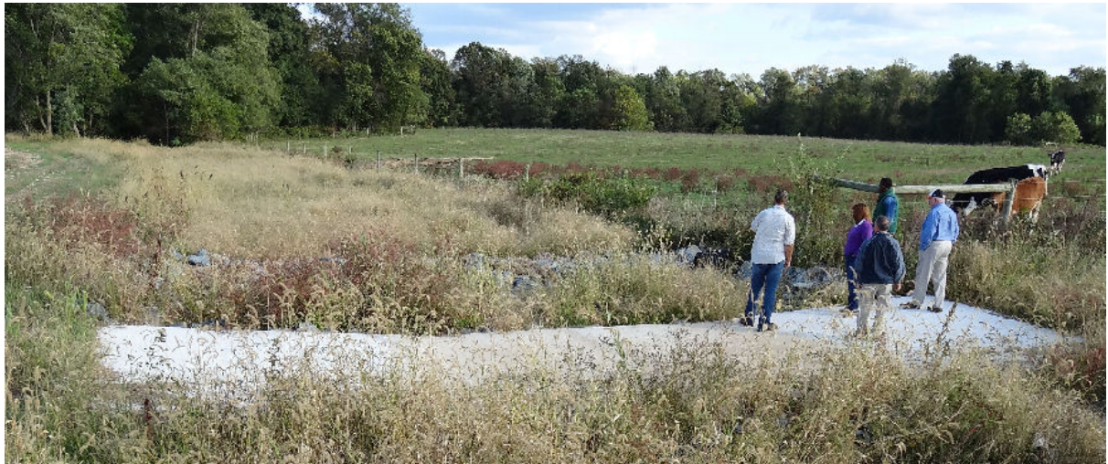
Figure 17. In mid October 2015 at the Phipps dairy farm in Kent County, Maryland, representatives of the Sassafras River Association and Kent Soil Conservation District are explaining the design of recently installed treatment wetlands to visiting MDE and EPA representatives. At this site, stormwater from the dairy's heavy use area flows across a concrete apron and over an area stabilized by riprap before entering the constructed wetlands. After passing thru three treatment cells, stormwater exits at the tree line. In the wooded area, the project also helped to stabilize a pre-existing 30-foot deep ravine. (photos by MDE. Federal funds: 319 FFY13 project 8. State funds: Chesapeake and Atlantic Coastal Bays Trust Fund. )
