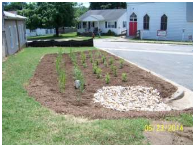
Figure 20. In the Town of Greensboro in Caroline County, a grassy slope adjacent to the Town Hall parking was identified in 2013 as a future bioretention site (top left). By June 2014, the installation of the project was just recently completed (bottom left). Then in October 2015 when EPA and MDE representatives visited the site the vegetation had filled in and the site was functioning as designed to capture and infiltrate parking lot stormwater runoff (bottom right). This project was one of several in Greensboro that used FFY2012 319(h) Grant funds to help implementation the Upper Choptank River Watershed Plan. (photos courtesy of Caroline County and MDE).
