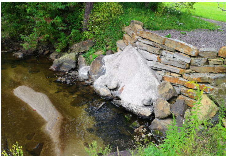
Figure 10. The site pictured (left) was installed on private land in 2015 to allow a delivery truck to backup adjacent to the stream and dump limestone “sand” stream at the stream edge. The limestone, which was crushed to the approximate size of sand particles, is allowed to wash downstream. In the stream, the limestone particles balance the low pH acid mine drainage water and to add buffering capacity in the stream. (photo by MDE Land Management Administration, Abandoned Mine Land Division.)
