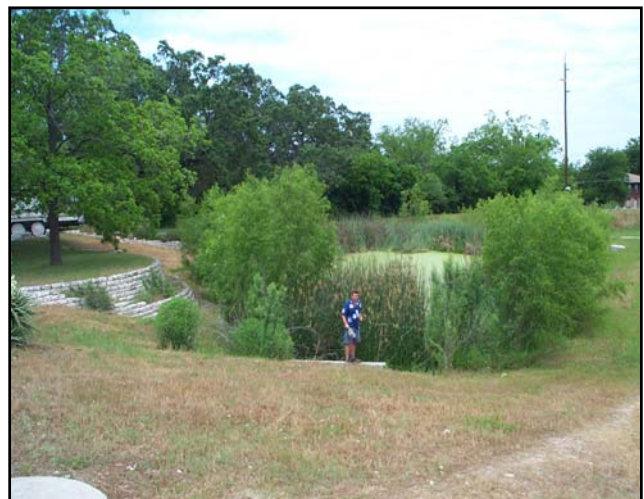
Figure 1: Warm temperatures have led to algal blooms in this wet pond.
