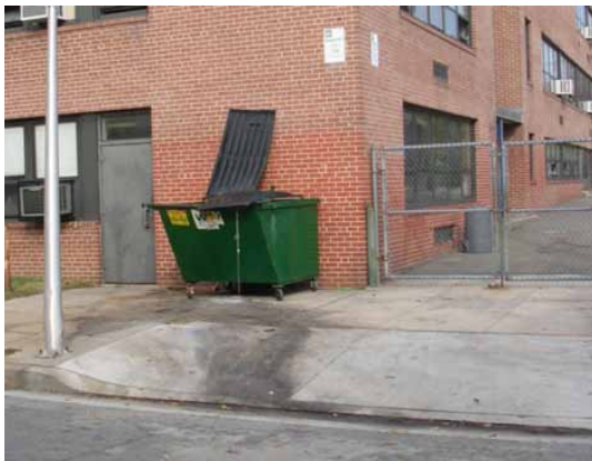
Staining from dumpster leading to storm drain at ISI site H-207
