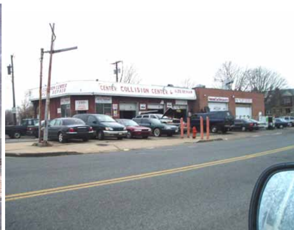
HSI site H-401, an auto shop where vehicles are repaired and stored outside
