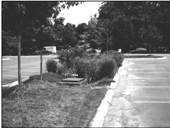
Figure 2: Parking Lot Island Turned Bioretention Area
