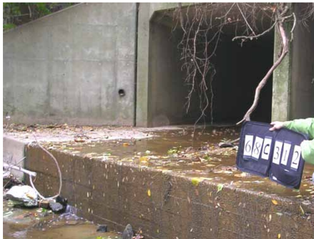
Site 68C312, a fish barrier downstream of a road crossing
