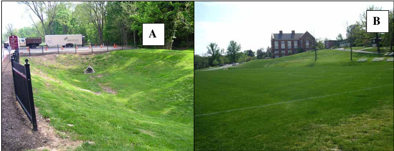
Figure 4.13. Opportunities at Boy's Latin School: A. Dry Pond for Planting or Conversion to Bioretention B. High Input Turf at College of Notre Dame.
