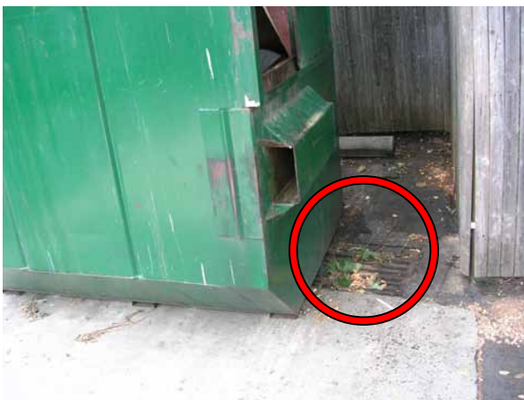
Dumpster juice” has direct access to the storm drain
