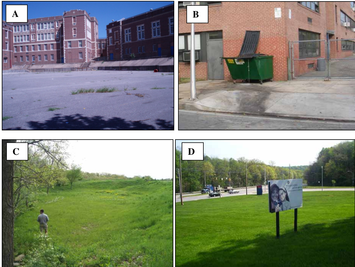
Figure 4.6. A. Extensive Impervious Cover Removal was Identified at Robert Pool Middle School and High School (ISI_H_206). B. Trash Management was Identified as a Necessary Pollution Prevention Practice at Waverly Middle School (ISI_H_207). Several Restoration Opportunities Identified at Sinai Hospital (ISI_H_200) include C. Retrofitting the Existing Dry Pond and D. Tree Planting in Pervious Areas.
