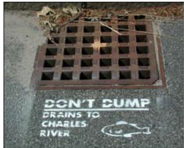
Figure 1: Storm Drain Marking
