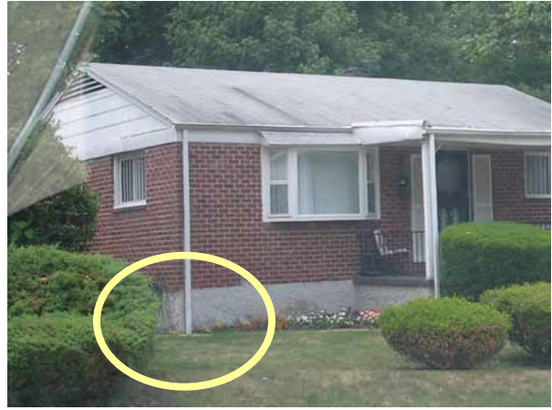
Directly connected downspouts in NSA-H-98A
