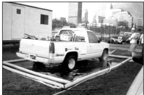
Figure 1: Containment System Preventing Wash Water from Entering the Storm Drain
