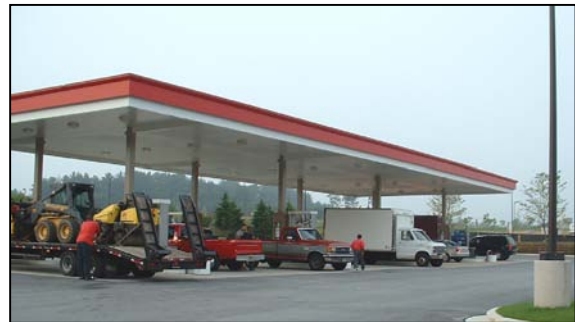
Figure 1: Covered Retail Gas Operation Without Containment for Potential Spills
