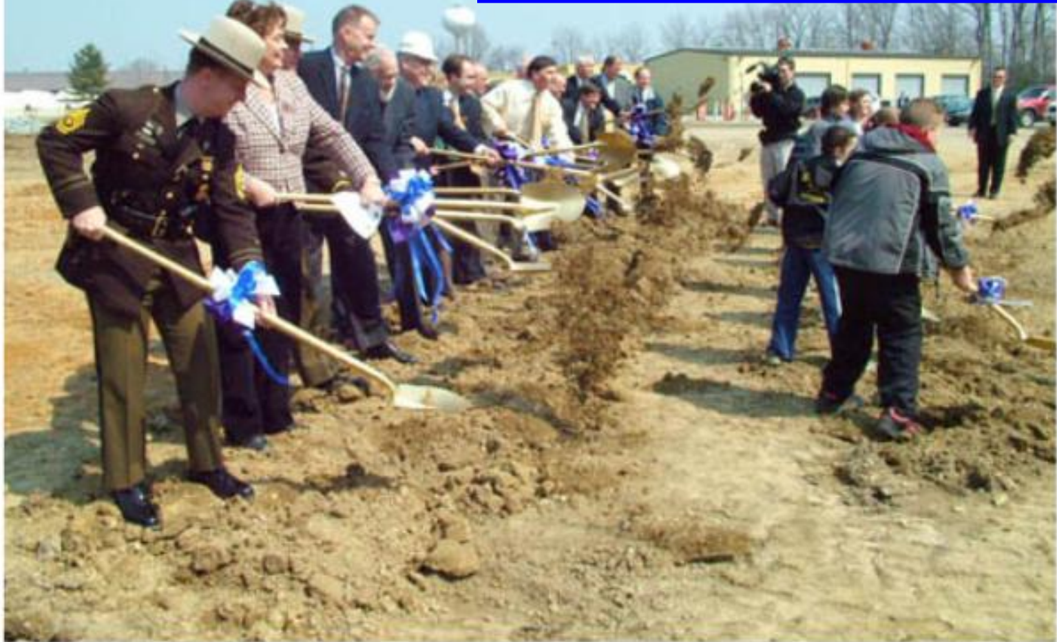
Ground breaking ceremony to kick-off construction to upgrade Kent Narrows/Stevensville/Grasonville Wastewater Treatment Plant on March 18, 2005.
