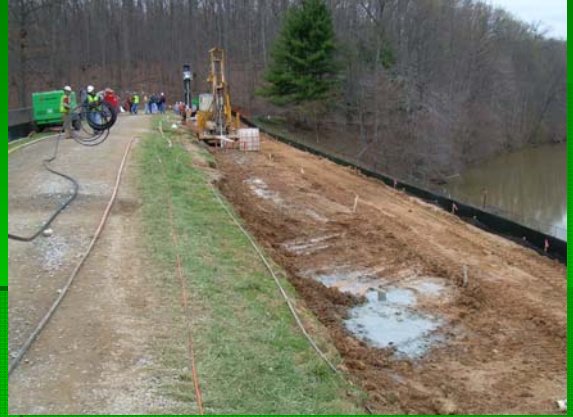
Grouting Work on Lake Needwood Dam
