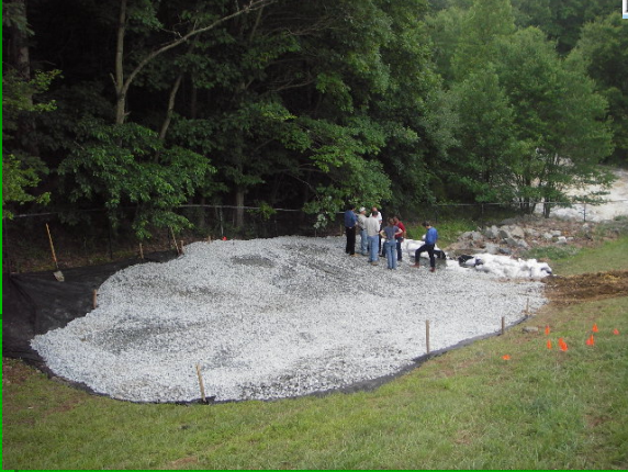
Seepage on DS Slope at Lake Needwood Dam
