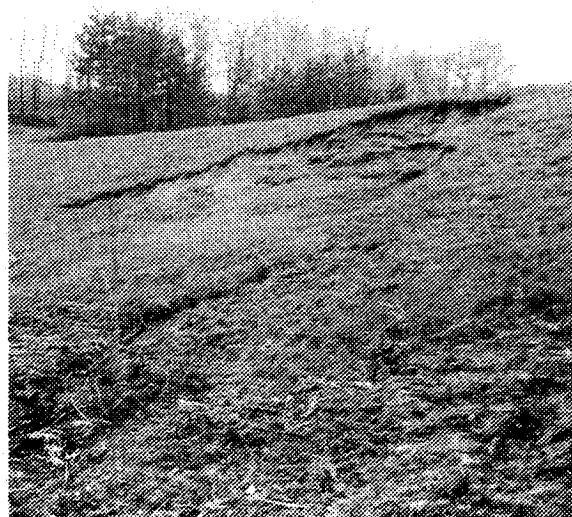
Slide Failure
