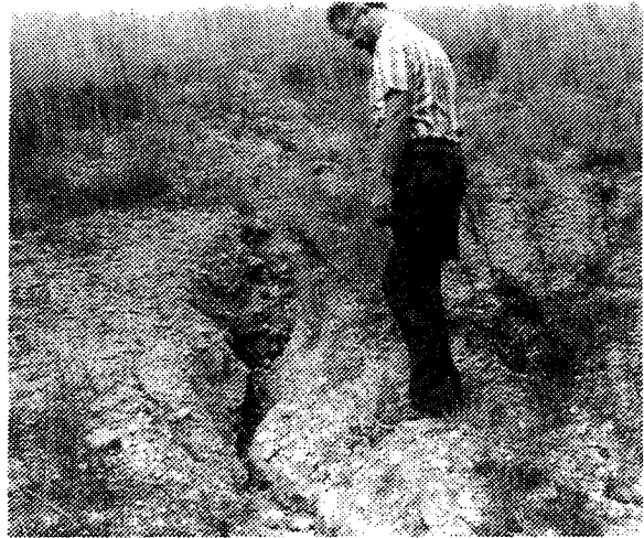
Erosion Left Unattended
