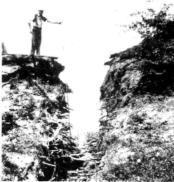
Failure Due to Root System
