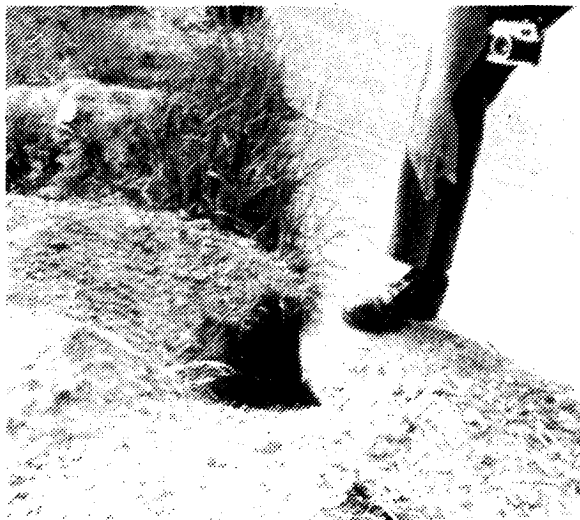
Burrow Under Slab
