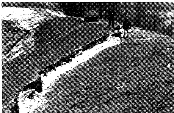
Transverse Crack
