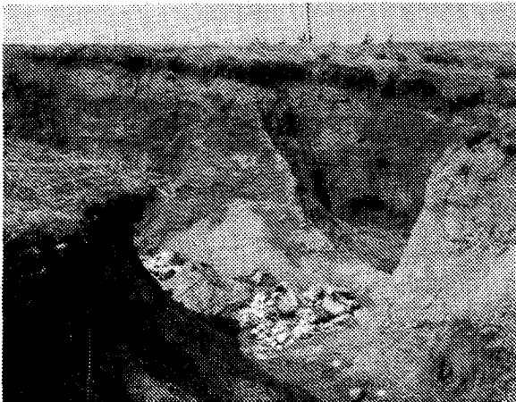
Eroded Spillway
