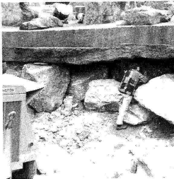
Erosion Under Outlet Slab
