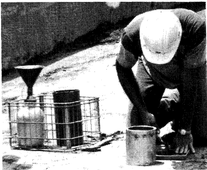
Testing Embankment Compaction
