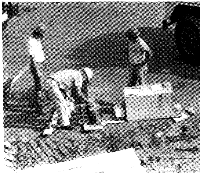
Testing Concrete Quality
