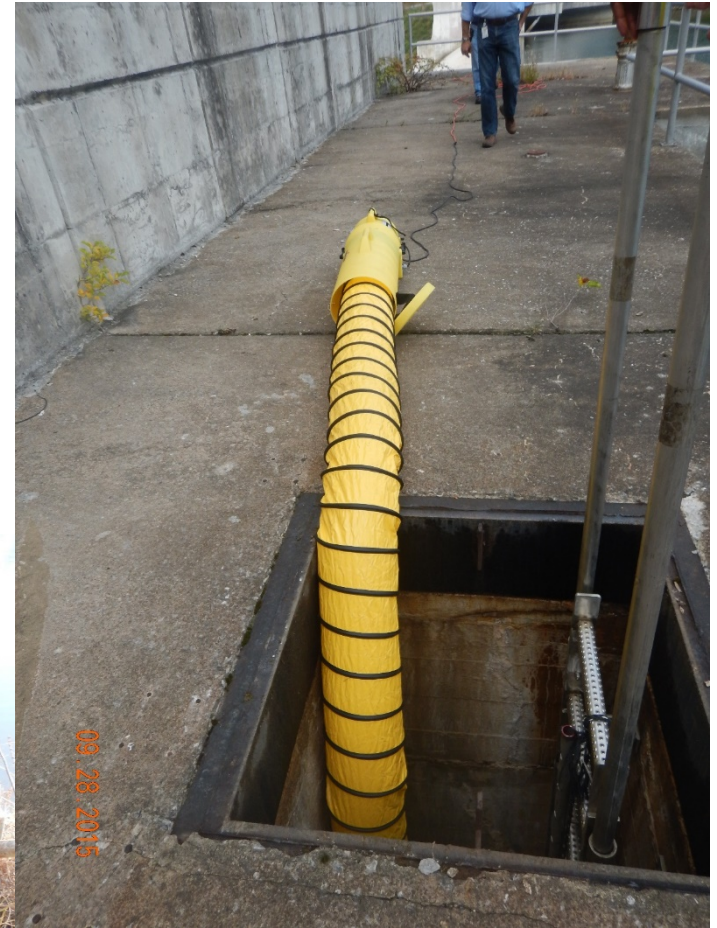
MDE File Photos: Loch Raven Dam, Baltimore City, MD.
