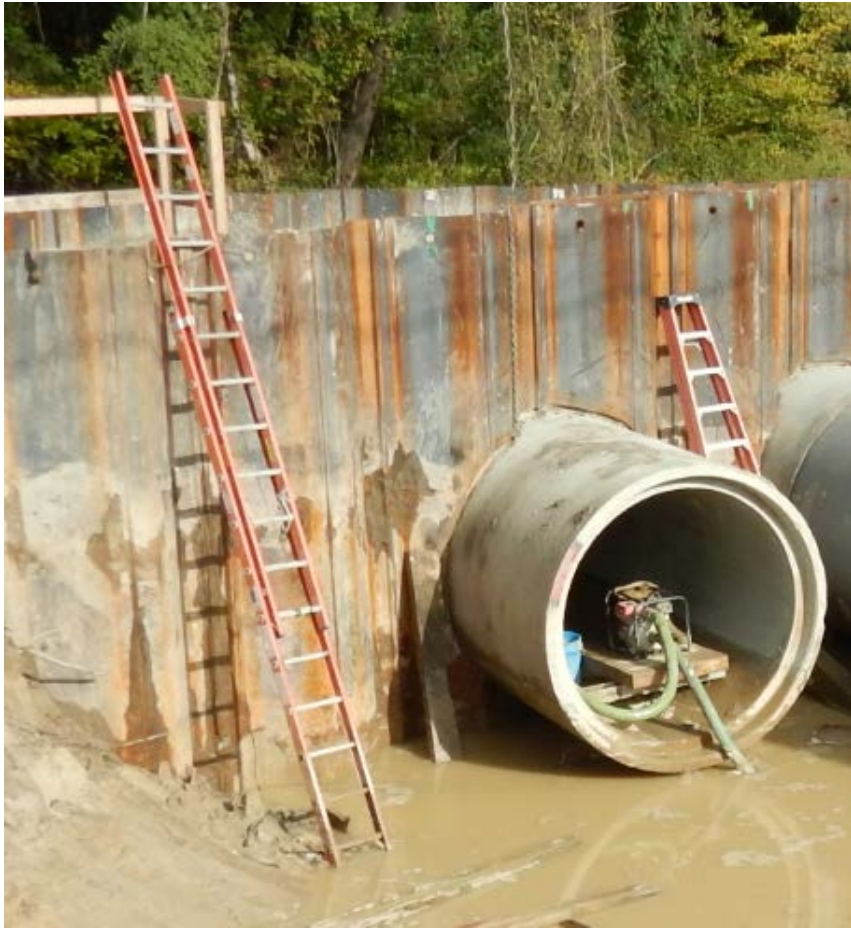
MDE File Photos: Morris Mill Dam, Salisbury, MD.
