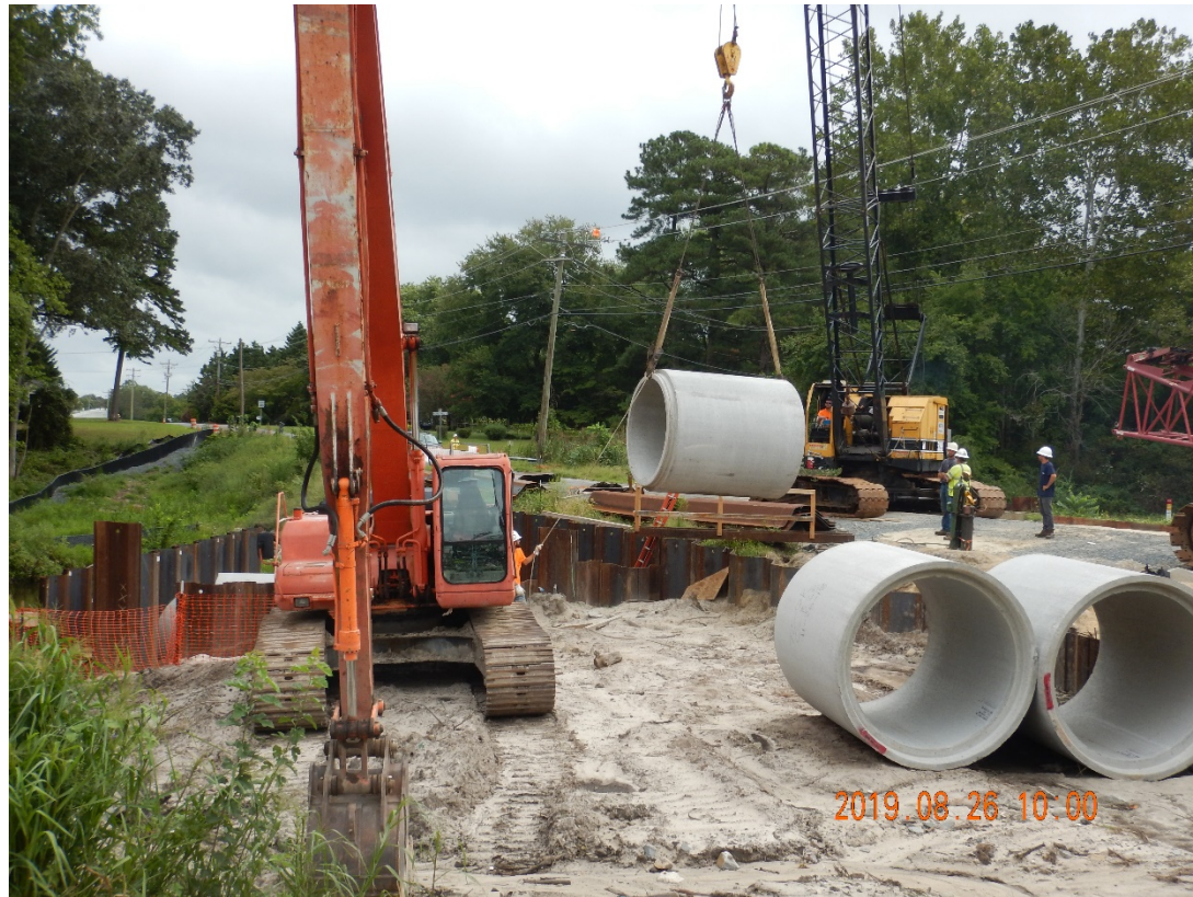
MDE File Photos: Morris Mill Dam, Salisbury, MD.
