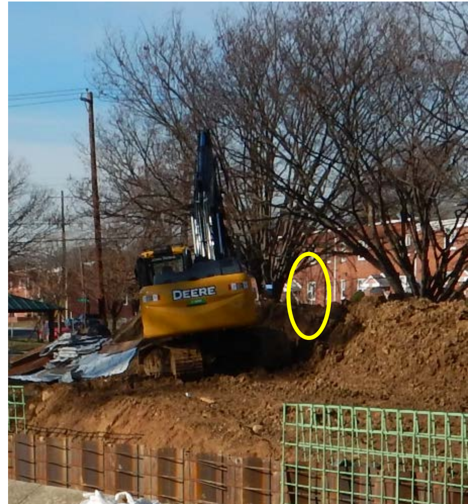
MDE File Photos: Allison Street Levee, Prince George's County, MD.
