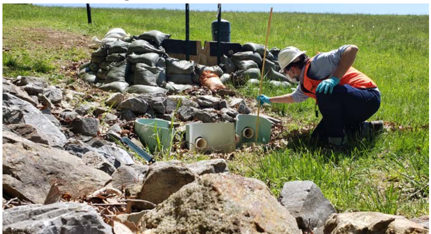
Socially Distant Inspector: Probing drain outfalls following another seepage incident at Greenbrier Dam
