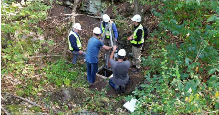
Confined Space entry protocols are required at an inspection vault. Savage River Dam
