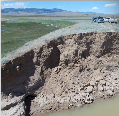
King No. 1 Dam – Wyoming
