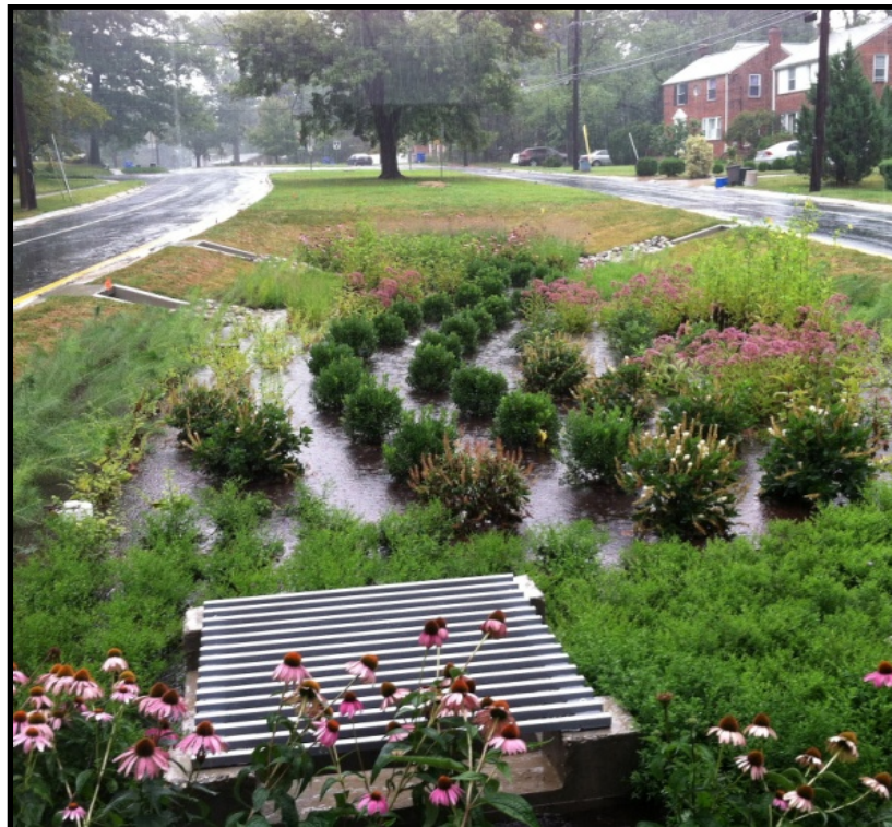
Figure 13: Bioretention, Denis Avenue Green Streets
