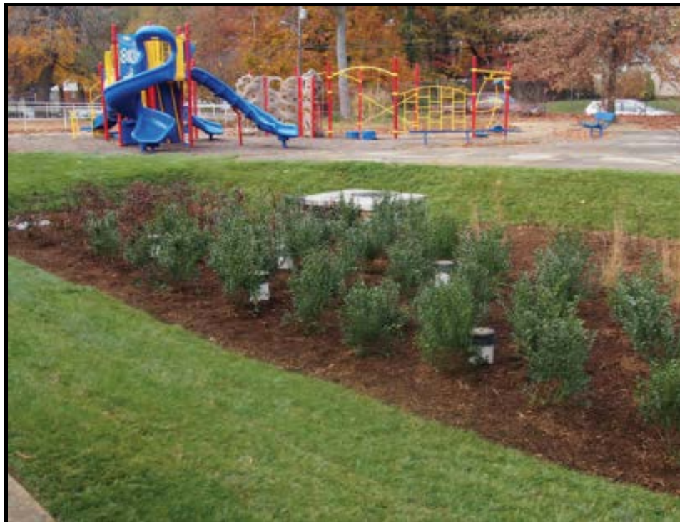
Figure 14: ESD Practice Installed Through the Partnership (Clean Water Partnership)
