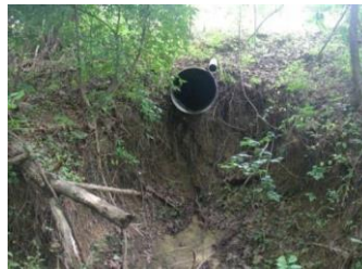
Figure B.1. The above outfalls are examples of locations that should be identified on storm drain maps and included in the permittee's screening program if they discharge to waters of the U.S. Areas with highly developed land uses (e.g., commercial business complexes, aging infrastructure) have a greater potential to pollute and should be prioritized. Structural stability and erosion concerns should also be identified and corrected as part of an
