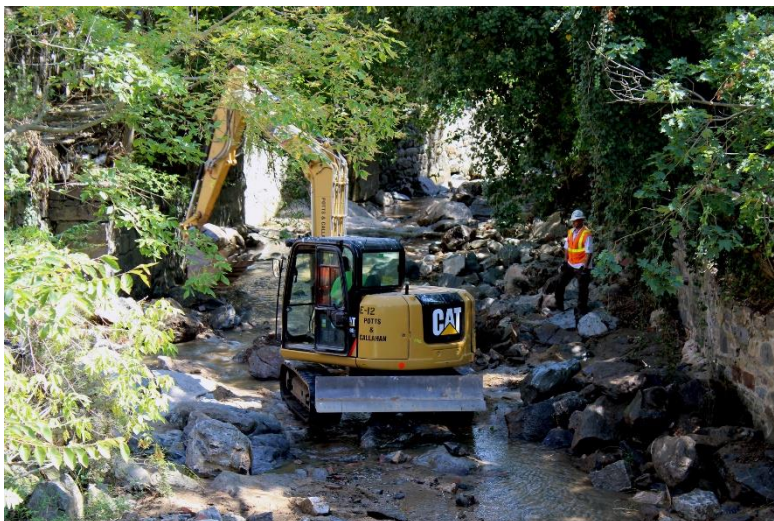
More than 50 cities and towns in the Chesapeake Bay watershed have antiquated, combined sewage and stormwater systems in need of major overhaul.
