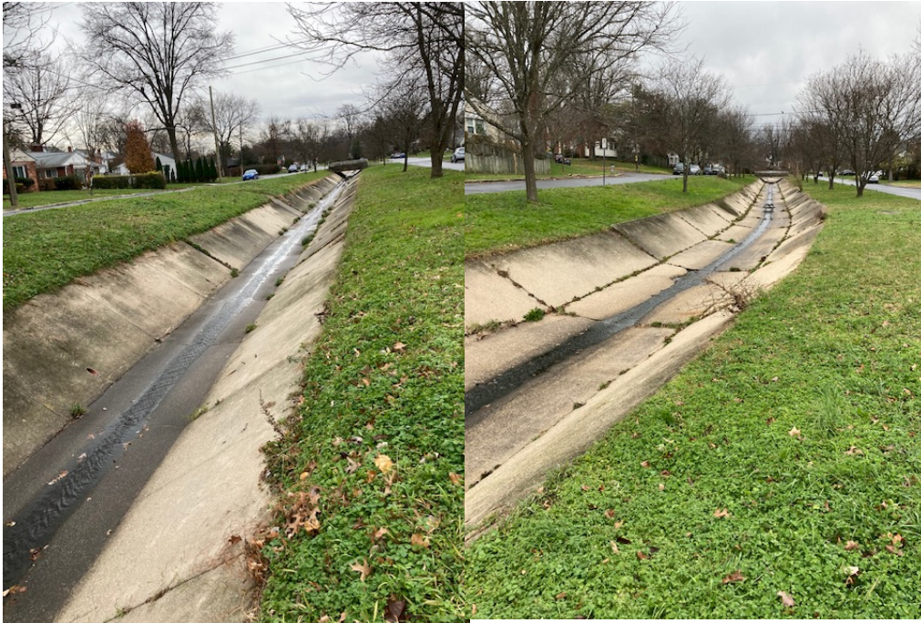
Figure 1. Concrete channel along Bucknell Drive.
