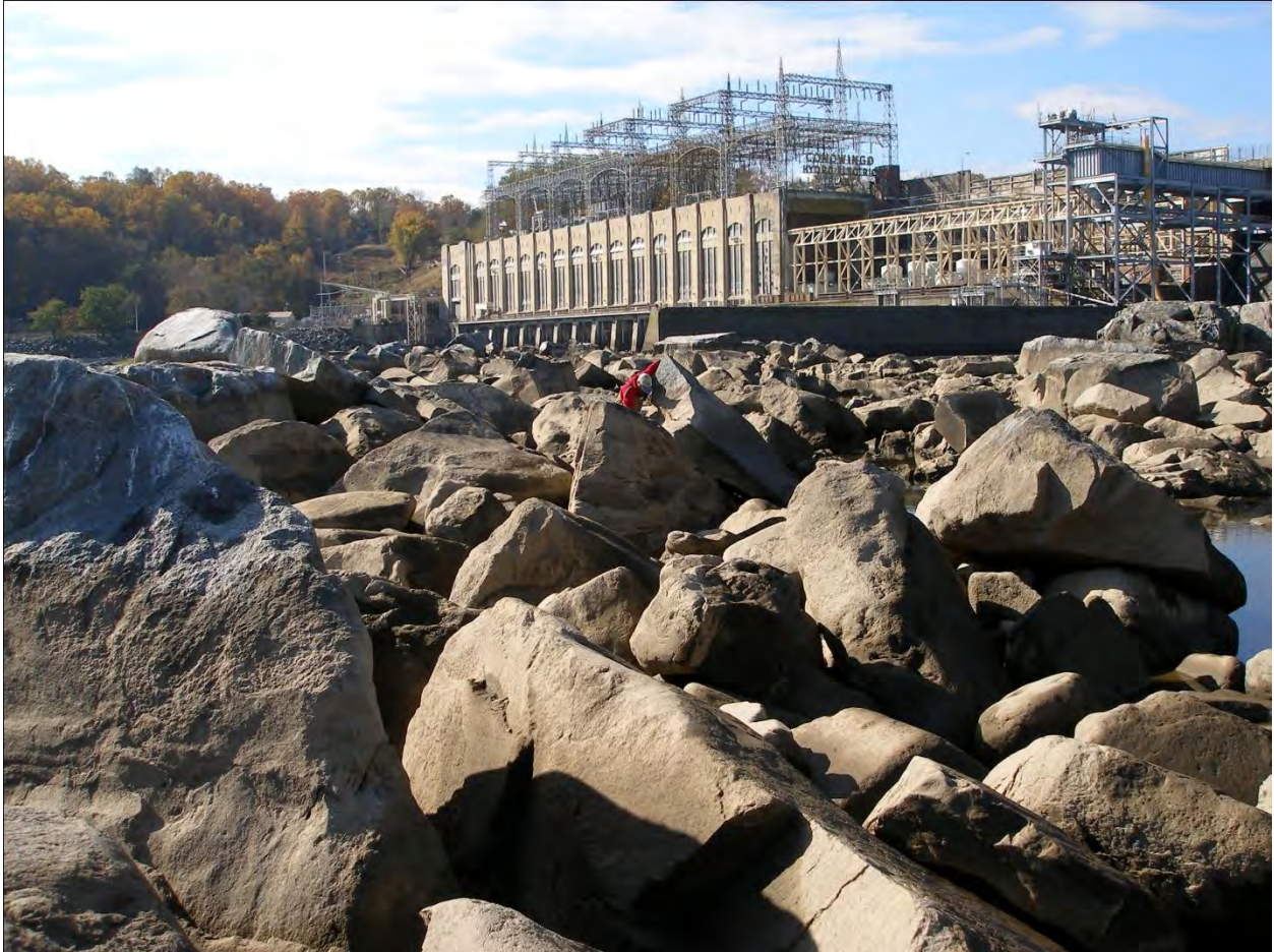
FIGURE 2-3: HIGH-RELIEF SPILLWAY REACH HABITAT.
