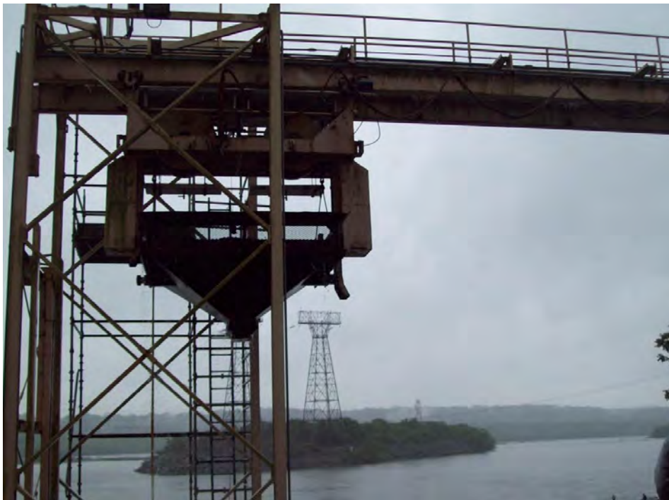
Photo 4. West Lift hopper in full up position, starting to travel along rail.
