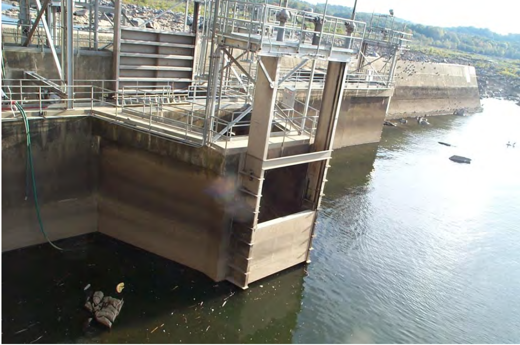
Photo 9. East Fish Lift, Weir Gate "A".
