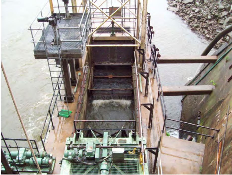
Photo 3. West Lift hopper starting a lift, looking downstream.
