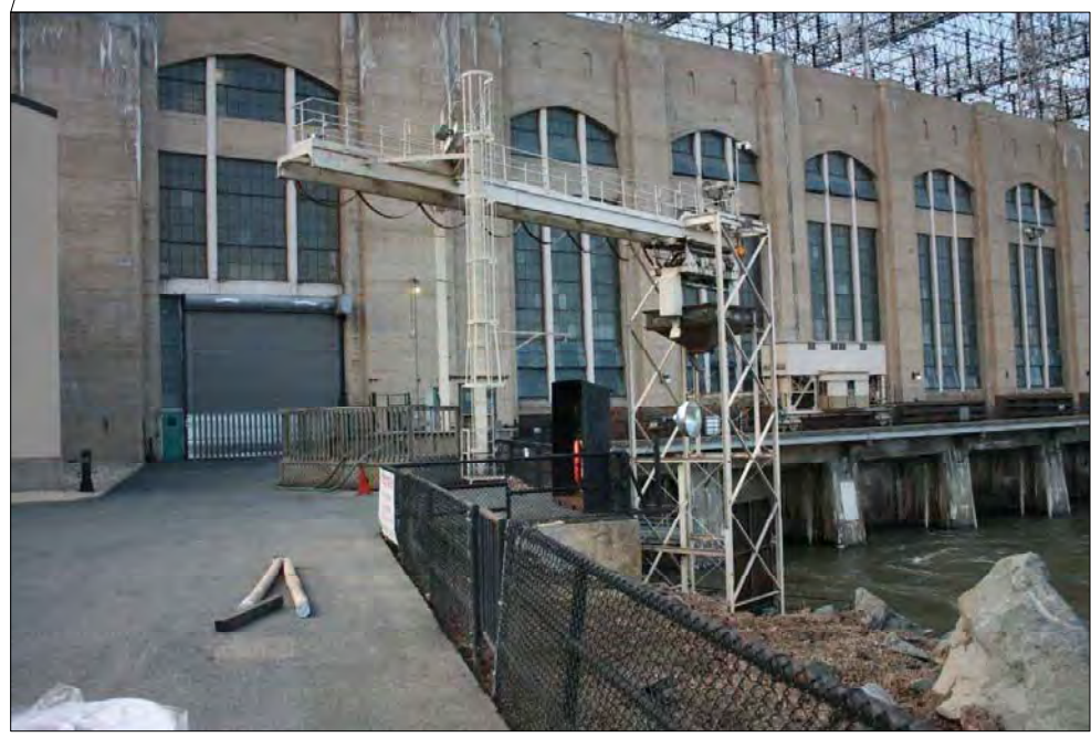
WEST FISH LIFT, AS VIEWED FROM WEST BANK.
