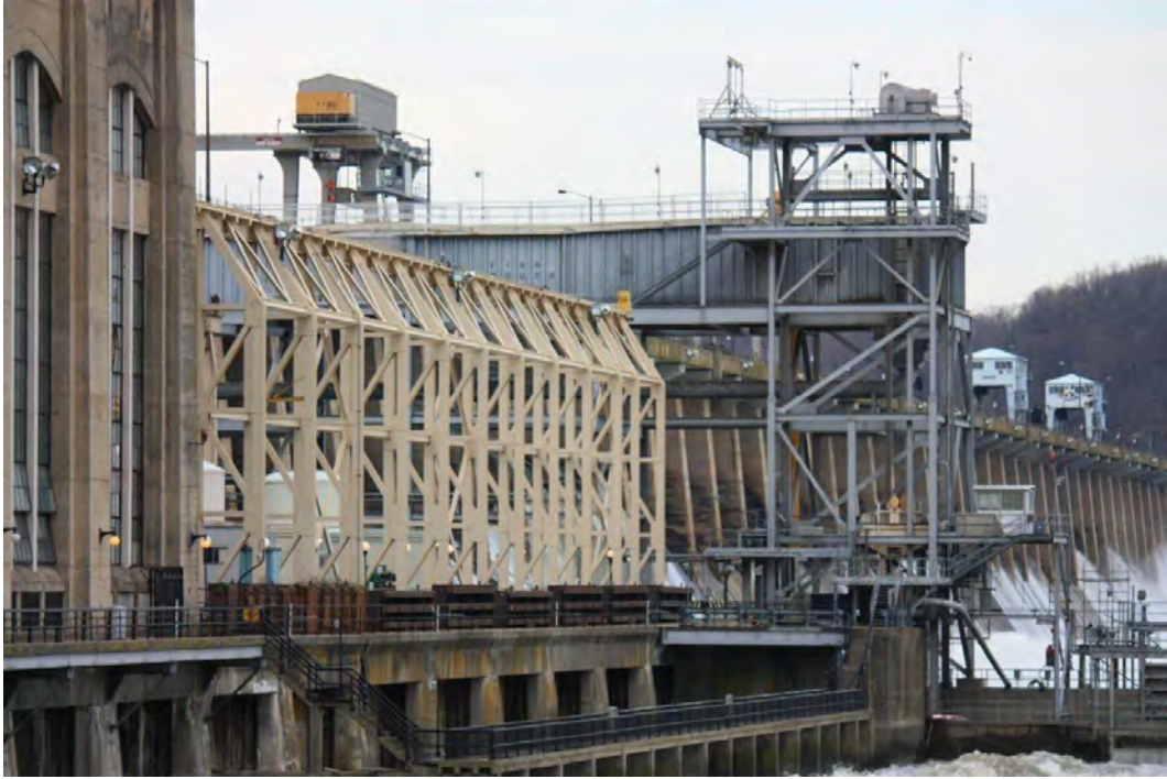
Photo 13. East Lift superstructure as viewed from west bank.
