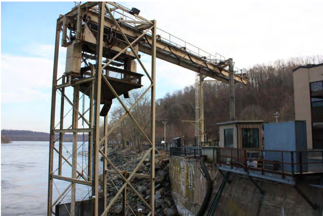
Photo 2. West Lift superstructure and hopper, as viewed from upstream side.
