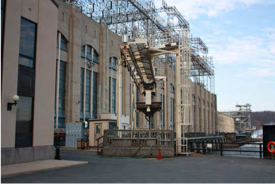
Photo 5. West Lift hopper and transport rail.
