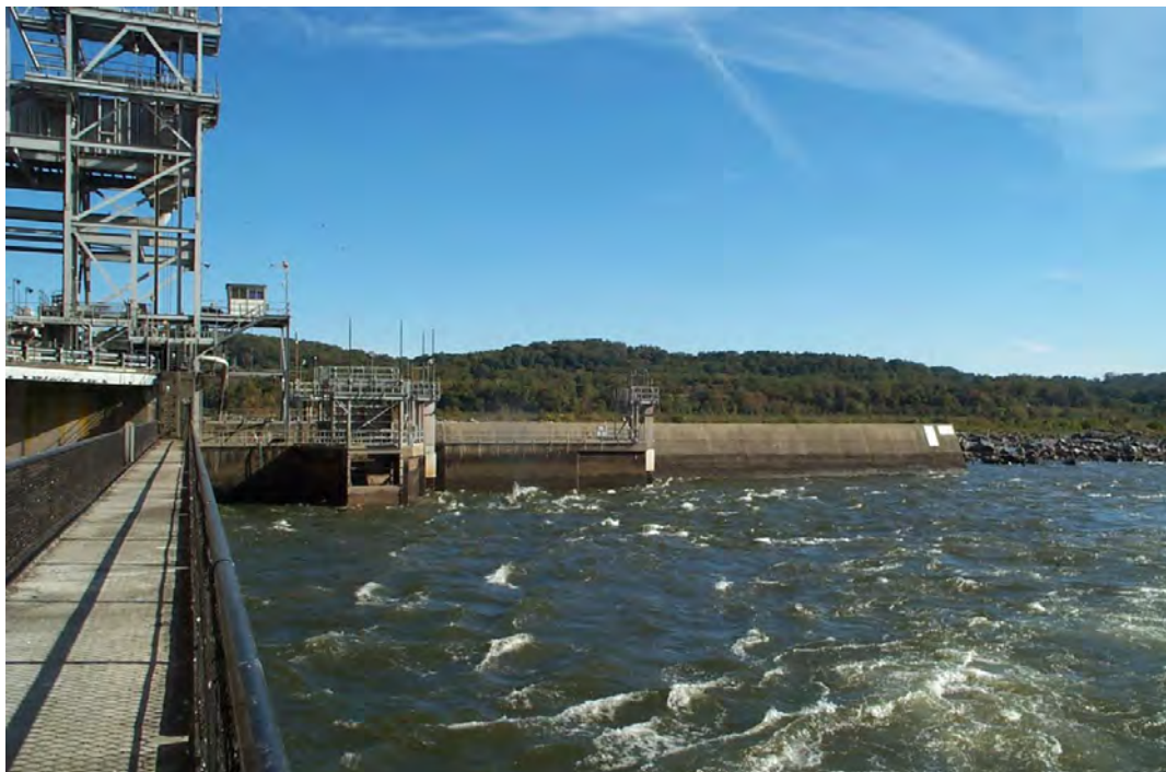
Photo 8. East Lift, looking east from downstream side of Powerhouse.
