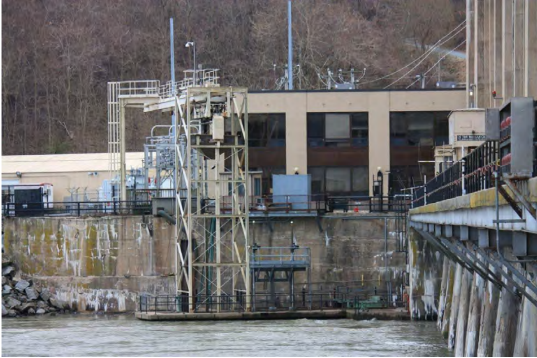
Photo 1. West Fish Lift, as viewed looking west from downstream side of powerhouse.
