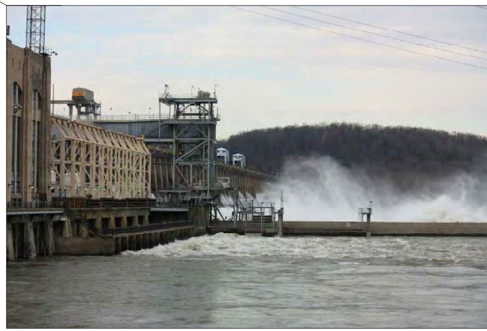
EAST FISH LIFT, AS VIEWED FROM WEST BANK.
