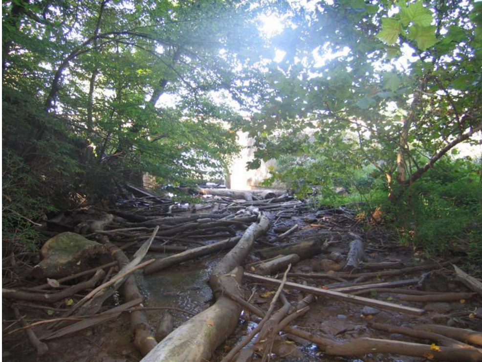
FIGURE 4.3-3: DEBRIS WITHIN TRIBUTARY. RAILROAD CULVERT IN BACKGROUND (SEPT 2007)
