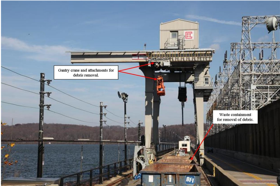
FIGURE 4.4.1-1: DEBRIS REMOVAL EQUIPMENT USED AT CONOWINGO DAM
