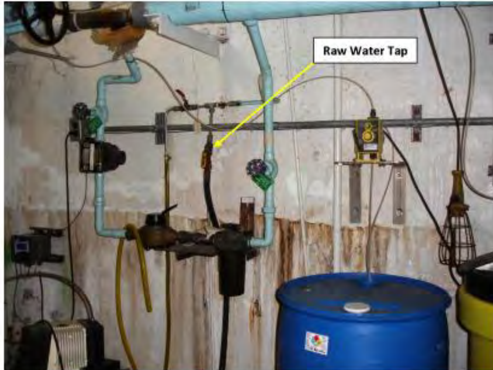
FIGURE 4-1: TOP PHOTO INDICATES THE RAW WATER TAP THAT WAS UTILIZED DURING SAMPLING EVENTS; BOTTOM PHOTO DEPICTS TYPICAL SET-UP FOR COLLECTING DREISSENID MUSSEL VELIGER THROUGH A 63 \mu MESH NET AT CONOWINGO DAM, APRIL THROUGH NOVEMBER, 2010.
