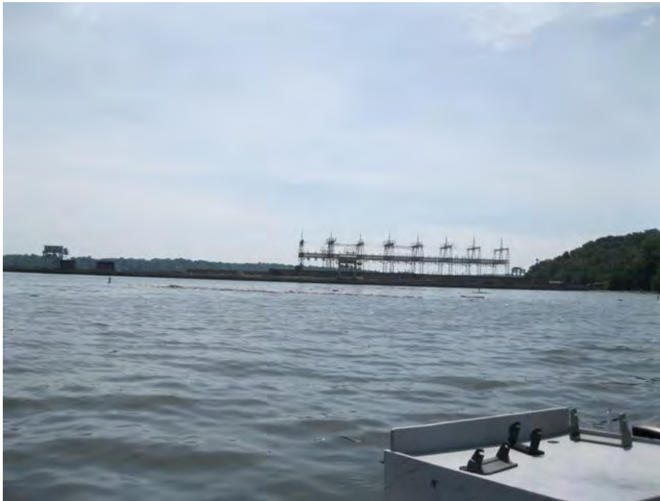
Photo 2: Conowingo Dam and superstructure viewed from upstream
