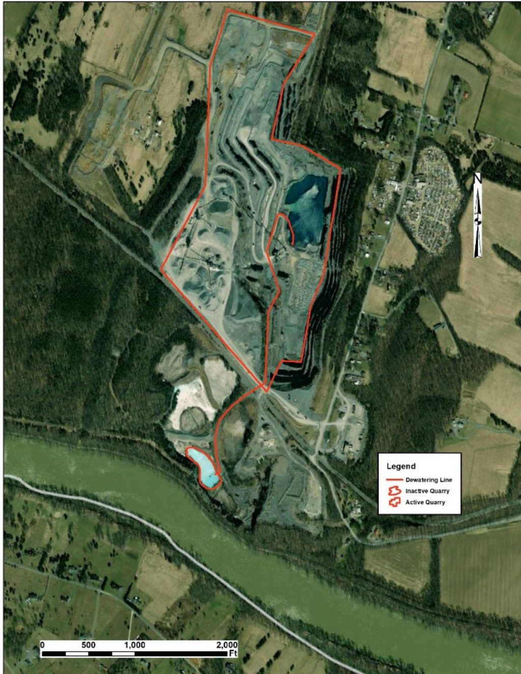
Figure 30. Aerial view of the Pinesburg Quarry showing dewatering line from the active quarry sump to the inactive quarry pond.
